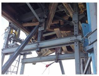
The lifting structures supporting the upper suspended part of the church were re-mounted
