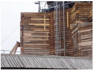
Tightening of annexes walls with cord strainers and wooden binding posts
